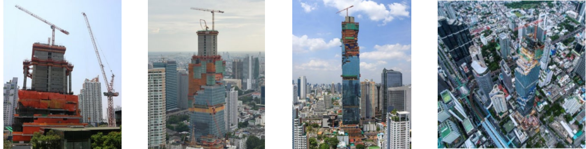
Image 2: COMANSA Cranes in the construction of the MahaNakhon tower in Thailand.
